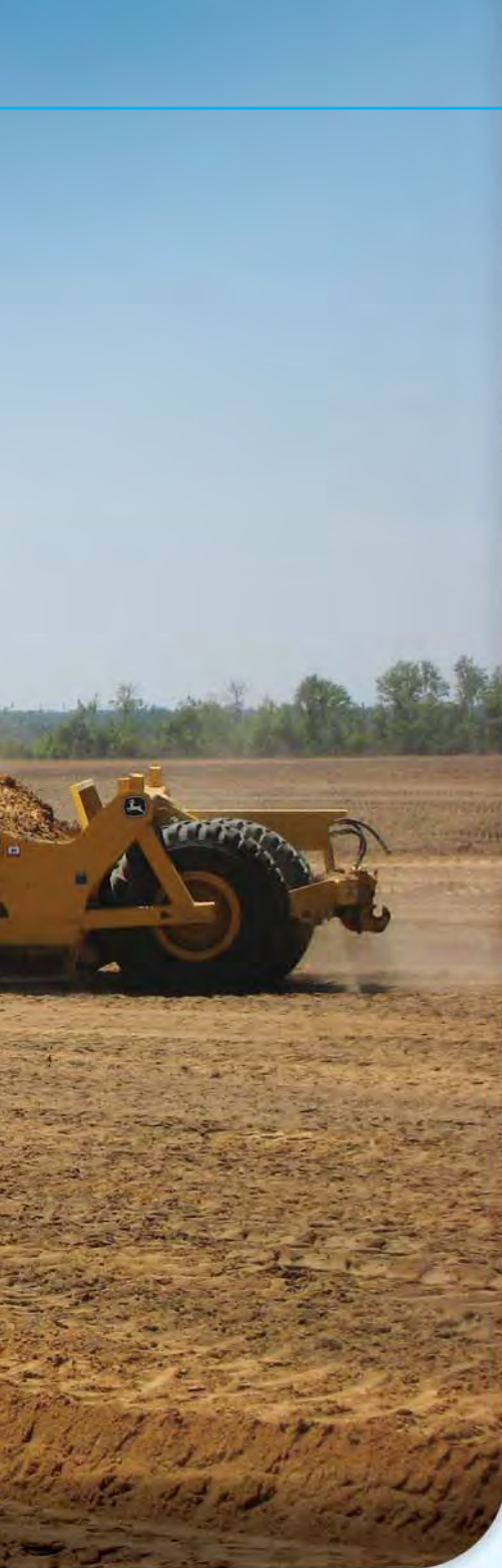
Above: Fig. 3. Initial stage of construction involved removing 12" of topsoil and stock-piling it.
