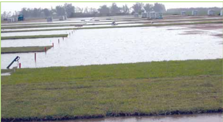
Fig. 2. The subgrade was laser-leveled and shaped to provide 5" drop from the outside inward to ensure all surface water flows to the center as evidenced during the rain event.
